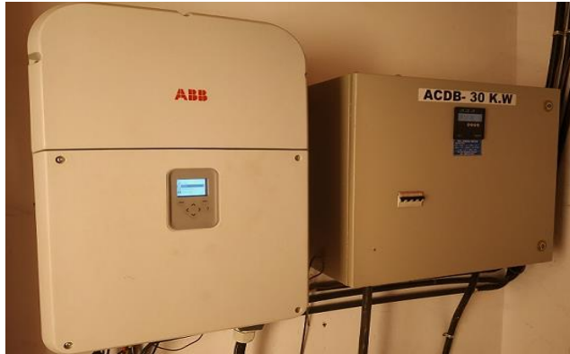
GRID TIED INVERTER & AC DISTRIBUTION BORD
